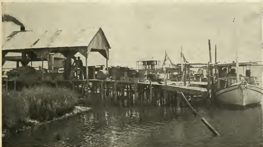
The brine-boiling tank of a shrimp sun-drying platform.
